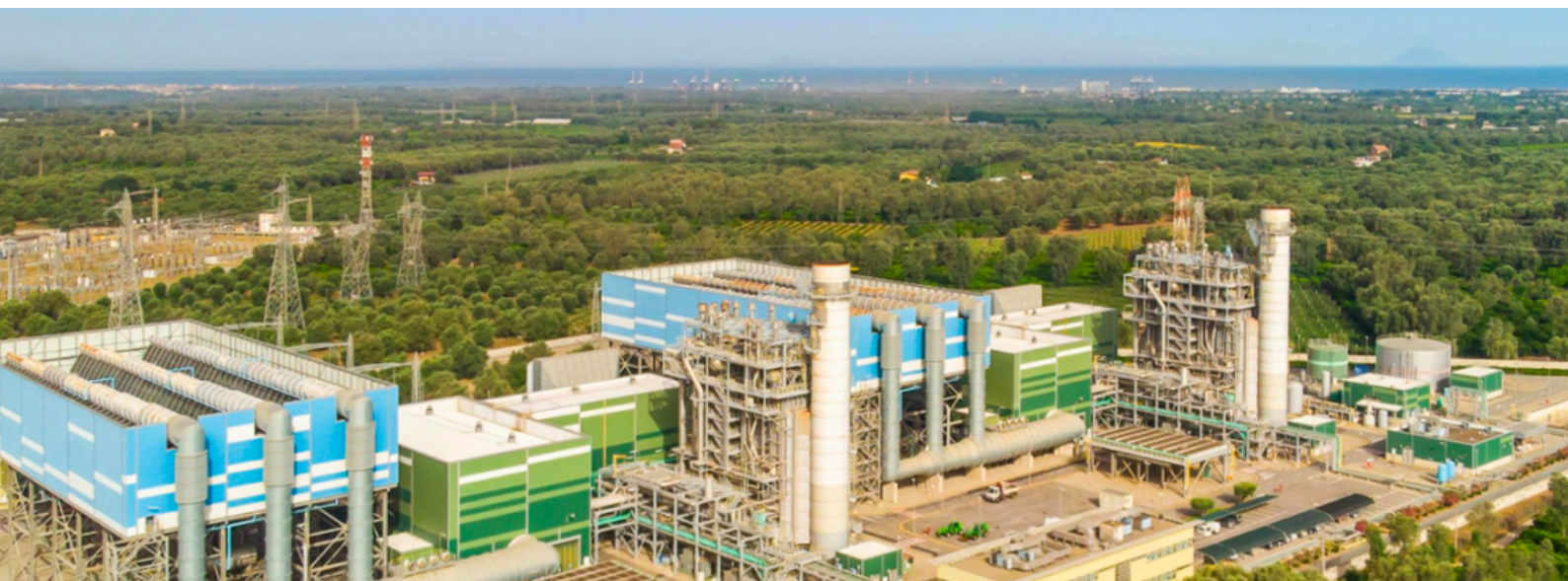
Figure 1: The plants at Rizziconi (shown here) and Sparanise are essentially twins and utilize two 1:1 combined cycle configuration consisting of a 260MW Ansaldo V94.3 gas turbine, a Heat Recover Steam Generator (HRSG), and a 120MW steam turbine. The cooling towers are within the blue structures, the turbines within the green structures, and the HRSGs are the tall structures adjacent to each exhaust stack.
