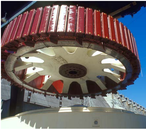
Figure 1: A hydro-generator rotor being lowered into its stator
