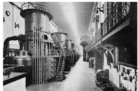
Figure 2: These vertical steam turbines were built by GE and installed at Chicago's Fisk Street Station in 1903. Each one produced 5MW – approximately 100 times more than the gas turbines of the era. It would be 1939 before the first gas turbine for power generation would be installed in the Eastern Hemisphere and 1949 before one was installed in the Western Hemisphere.
