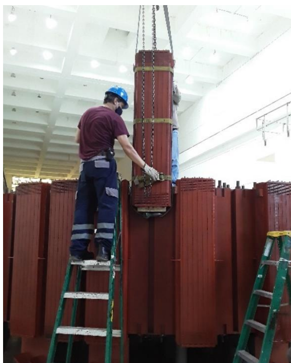
Fig. 13 : Insertion of poles of Unit No.1 in Cerrón Grande HPP, post maintenance and electrical tests performed on the repaired poles.
