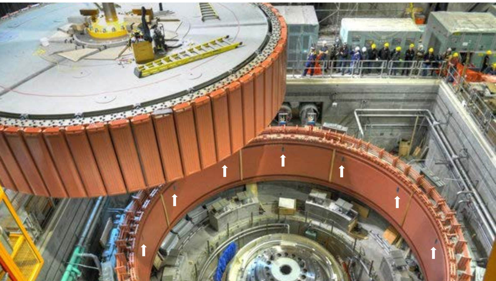
Figure 2: A hydro generator rotor being lowered into place. Note the relative size of the ladder atop the rotor and of the workers along the railings. Such massive sizes are quite common in many hydro plants where vertically oriented turbine-generator units are used. Note also the single layer of stator-mounted air gap sensors (seven are visible) as indicated by the white arrows.
