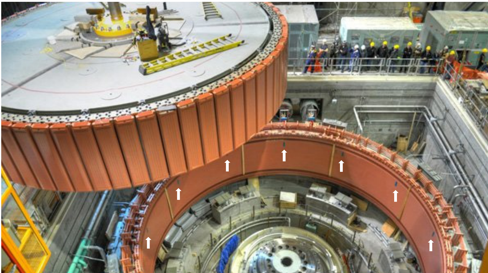
Figure 2: A hydro generator rotor being lowered into place. Note the relative size of the ladder atop the rotor and of the workers along the railings. Such massive sizes are quite common in many hydro plants where vertically oriented turbine-generator units are used. Note also the single layer of stator-mounted air gap sensors (seven are visible) as indicated by the white arrows.
