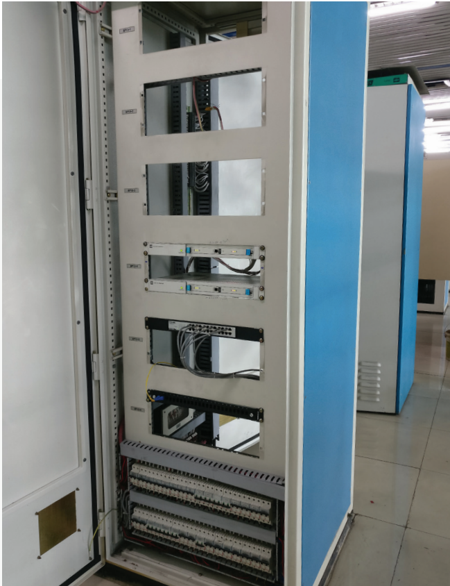
Figure 2: Two TSI racks are used to provide machinery protection for each unit and are visible in the left-most cabinet. These racks have been in service since the units were commissioned in the 2008-2010 timeframe. The adjacent cabinet to the right holds the condition monitoring hardware.
