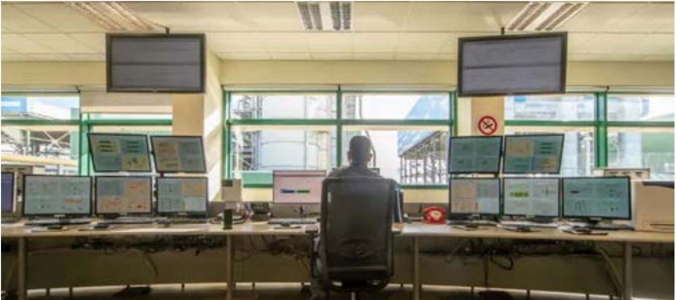
Figure 7: An operator at Rizziconi Energia keeps watch over the two 380MW combined cycle processes from a control room vantage point overlooking the plant.
