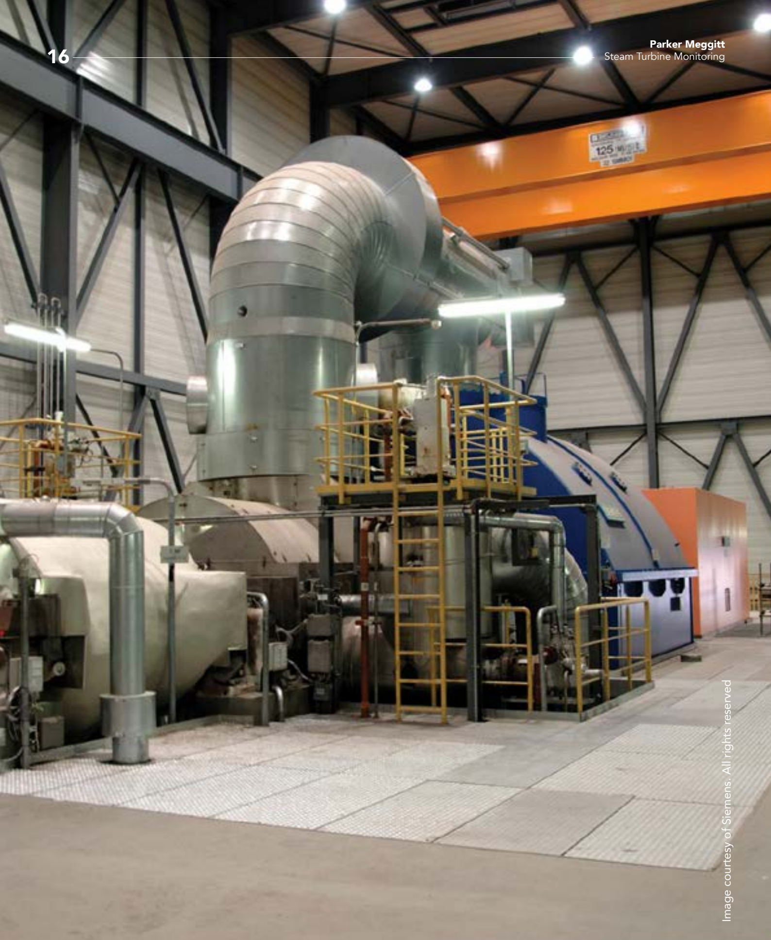
Figure 6: This 140MW steam turbine is used in a combined-cycle plant in Germany. Steam turbines in combined-cycle service have been specially enhanced over the last several decades to meet the demands of the steam conditions found in combined-cycle plants along with numerous other improvements 1 .
