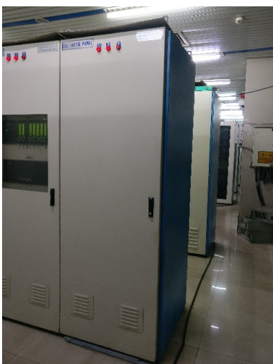
Figure 2: Two TSI racks are used to provide machinery protection for each unit and are visible in the left-most cabinet. These racks have been in service since the units were commissioned in the 2008-2010 timeframe. The adjacent cabinet to the right holds the condition monitoring hardware.
