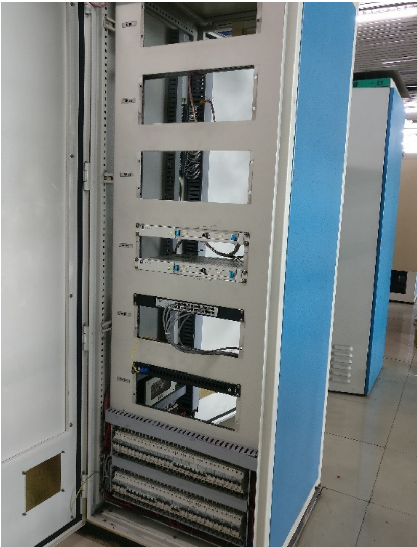
Figure 3: Cabinet from figure 2 but with door open showing vacated panel cutouts from old condition monitoring hardware. The incumbent CMS required six (6) large data acquisition units for each turbine generator and its accompanying boiler feedwater pumps (BFPs), as noted by the six panel cutouts. Note that the new vibro-meter data acquisition hardware for the turbine generator occupies only two-thirds of a single panel cutout (fourth opening from top) and thus consumes three times less space. Fitting the new CMS into existing panel space was an important project requirement as there was no room for any additional cabinets. The BFPs are slated to be added in a later project and will use a portion of the other cutouts.
